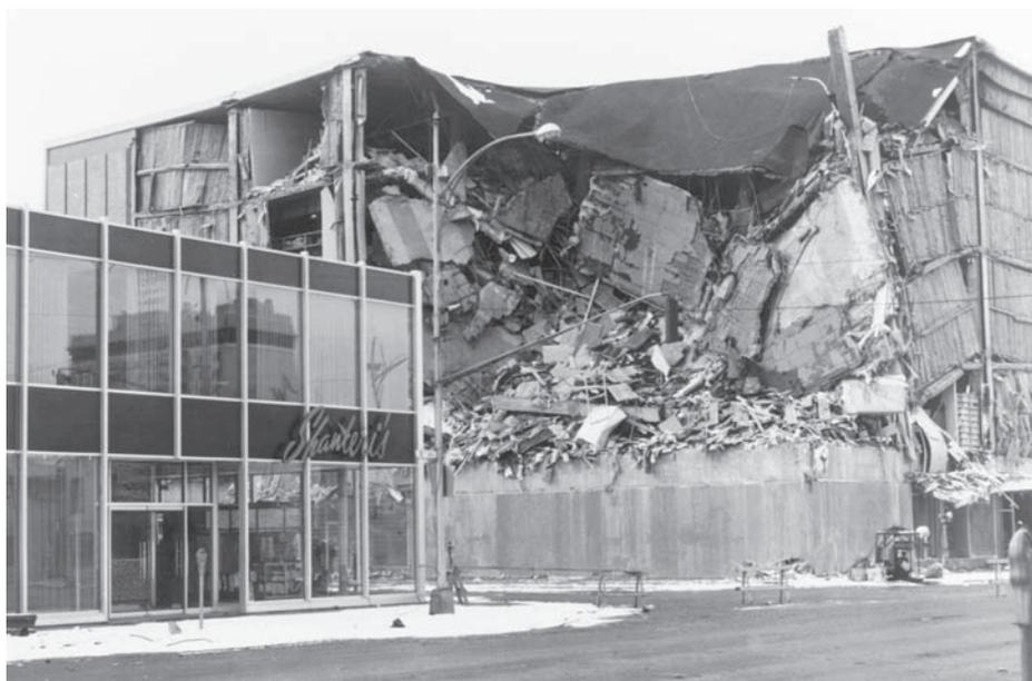
◆ **Figure 10.14** Damage caused to the five-storey J. C. Penney Co. building, Anchorage, Alaska. Very little structural damage was incurred by the adjacent building. (Courtesy of NOAA/Seattle)
