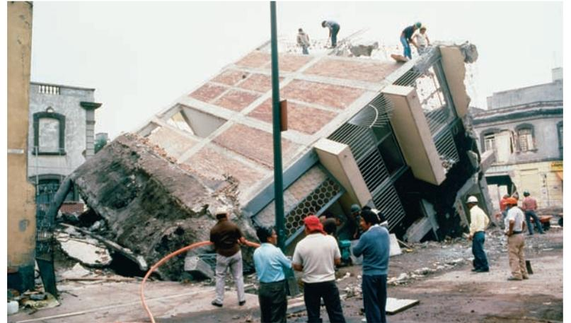
◆ **Figure 10.15** Effects of liquefaction. This tilted building rests on unconsolidated sediment that behaved like quicksand during the 1985 Mexican earthquake. (Photo by James L. Beck)
